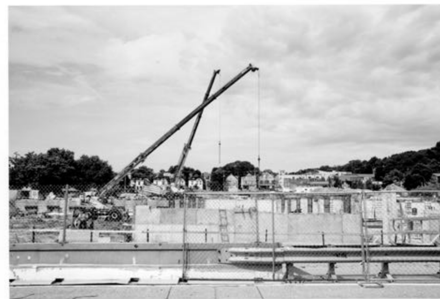
5704 Penn Ave. Former Penn Plaza Apartments
